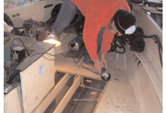
Steven, working on the deck.
